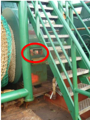
Figure 5: Emergency stop of the winch behind the stairs
